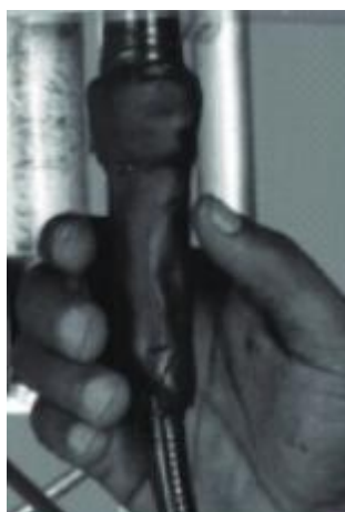
Figure 2-3 Wrapping Waterproof Clay
