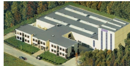
ASSMANN Hauptsitz, Deutschland ASSMANN Headquarter, Germany
